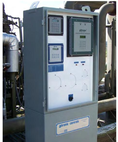
timing by a few degrees did the trick. This engine has been running with the ignition timing retarded due to the detonation problems and timing variations with the previous ignition system. With the new ignition timing, now set properly, fuel consumption was reduced but no on-site devices were available to determine the amount of reduction.
