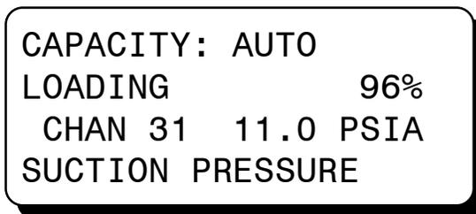
Indicates that the current value of channel 31 is above the desired setpoint by more than the allowable deadband and the output of the controller is being changed to increase the load, which will cause the suction pressure to decrease towards the setpoint.
