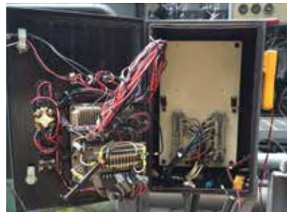
Wires have been disconnected; the ESCM is isolated and no longer a part of the system.
